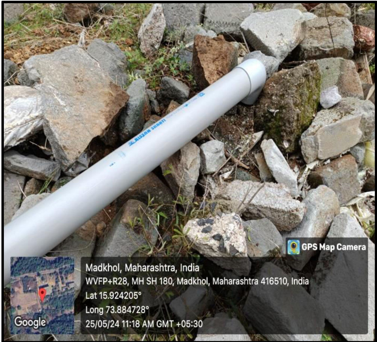
Rain water Harvesting pit
